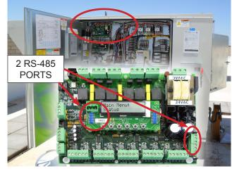
ager of the package it is controlling. The MicroMag provides flexibility with set points and control options that can be selected prior to commissioning a system or when the unit is live and functioning.
